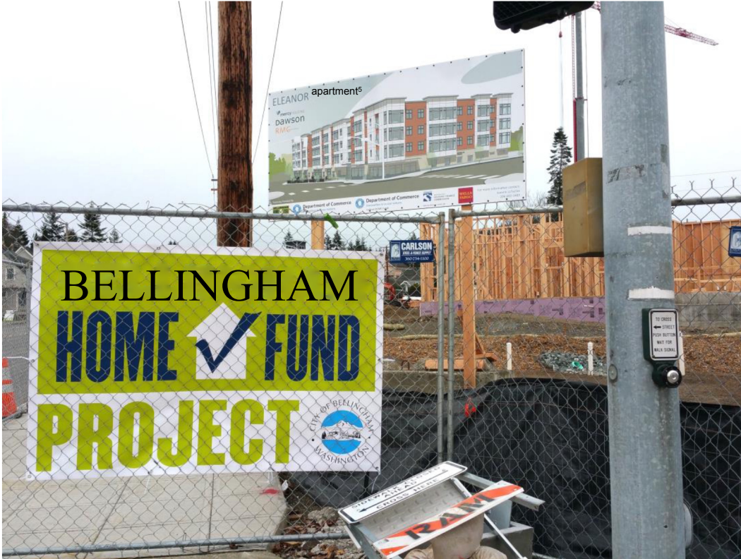
On Ellis St, new dense and affordable apartments are being built for low-income seniors. Good for the climate, good for people. (Galen Herz)
